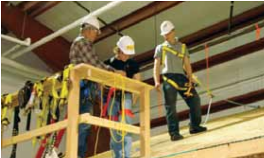
Top, senior CT students Vitaliy Kulinich and Yan Torba weld on the trailer project. Above, instructor Gary Hall, Craig Cummings, and Yan Torba at fall protection training.
