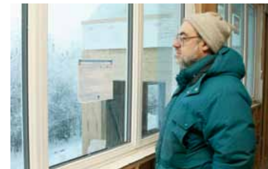
Extension Energy and Housing Specialist Rich Seifert reads a specification label on a recently installed energy-efficient window at the site of the Cold Climate Housing Research Center, currently being built on the UAF campus. CES photo by Jeff Fay
