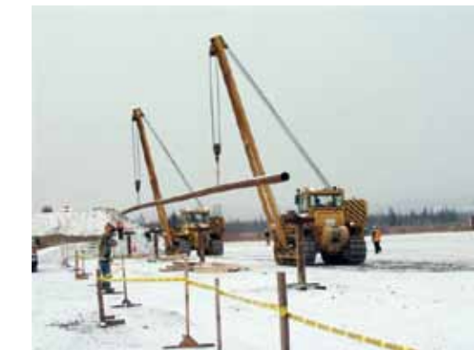
The fourth annual Alaska Pipeline Crafts Joint Training organized by Alaska Works Partnership in cooperation with Alaska's four pipeline unions culminates in a day of celebration during which trainees demonstrate what they have learned. Above on October 27, 2005 trainees demonstrate how side-boom tractors carefully lift pipe into position in slings guided by a worker at each end.
